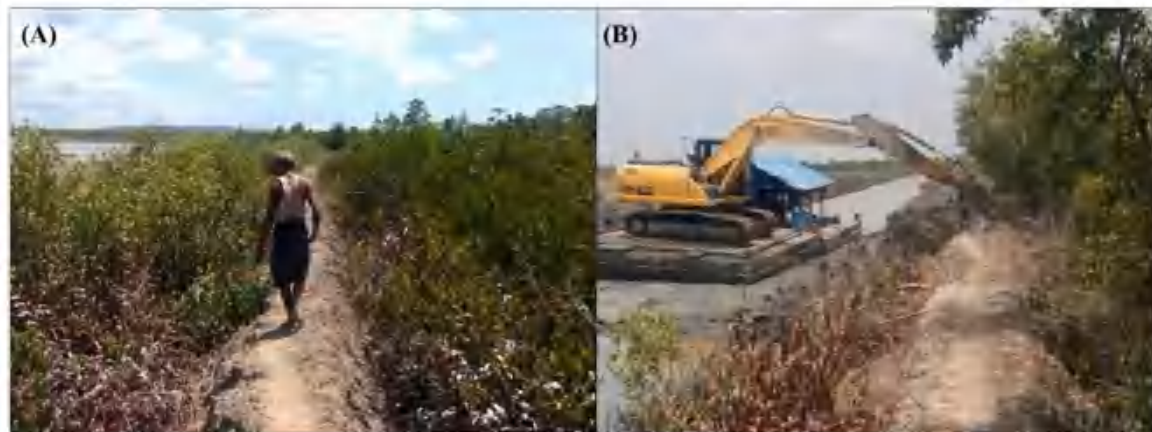
Fig. 11. Maintenance of a ~400-acre shrimp pond near the Kyaukpyu–Yangon Road (2017): (A) condition prior to rehabilitation; (B) rehabilitation/maintenance underway using heavy machinery.
