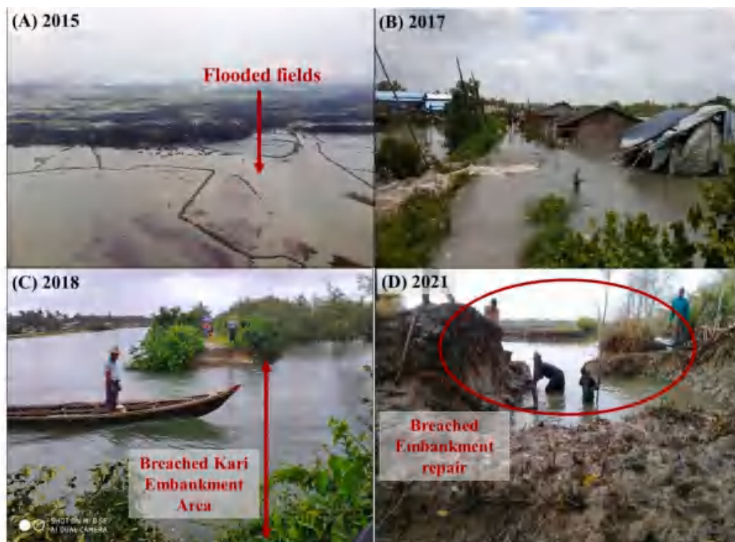
Fig. 12. Examples of coastal flooding and embankment (“Kari”) damage in Rakhine State and Kyaukpyu: (A) flooded fields in Rakhine following Tropical Cyclone Komen (July 2015; photo by FAO-Bu Thi Lan); (B) seawater entering through a breached embankment during an unusually high tide in Kyaukpyu (2017) (BBC, 2018); (C) breached Kari embankment in Kyaukpyu during high tide (Myanmar Now, 2018); and (D) local residents repairing storm-damaged Kari embankments after a tropical storm (Eleven, 2021).
